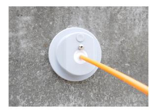
The Filoform MD1-FttH is designed for gas and watertight sealing of FttH home entries with micro ducts and cables.
